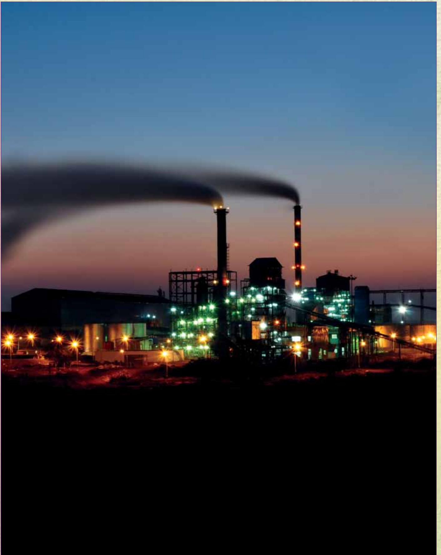
Night view of the whole plant
