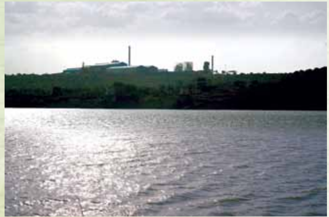
Dam side Location
